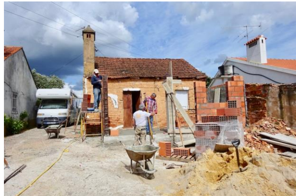
Floors levelled and walls going up.
