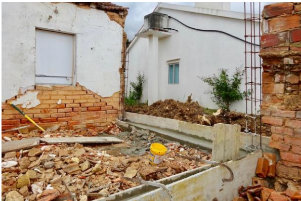
Old extension down and start of new.
