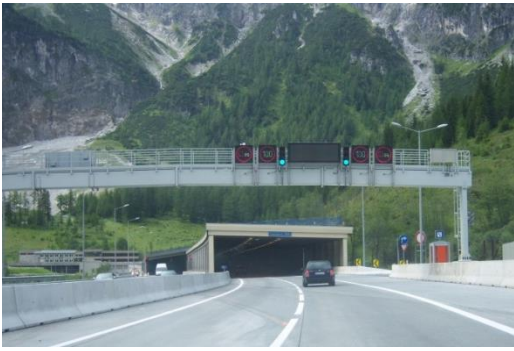
Approaching the Tauern Tunnel
